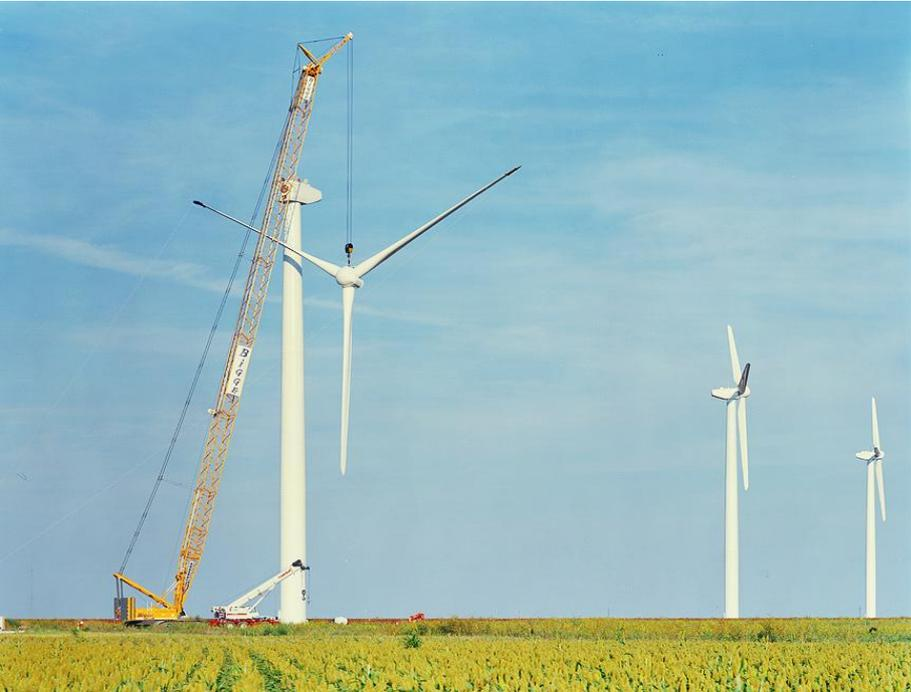
Fig 7: Crawler crane with Carbo-Link pendant cables with superior handling and fatigue life.
