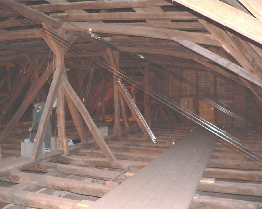
Fig 6: Repair of a 400 year old timber structure using Carbo-Link cables with load sensing devices
