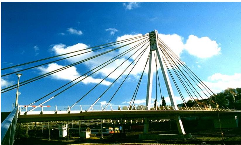
Fig. 3: First road bridge in the world with bundled carbon fibre cables built in 1996.
