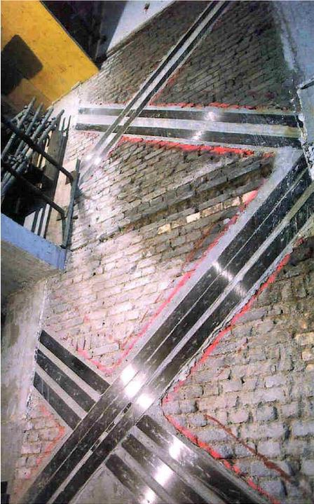
Fig 5: Shear strengthening of an existing masonry wall with externally bonded carbon fibre ribbon cables.
