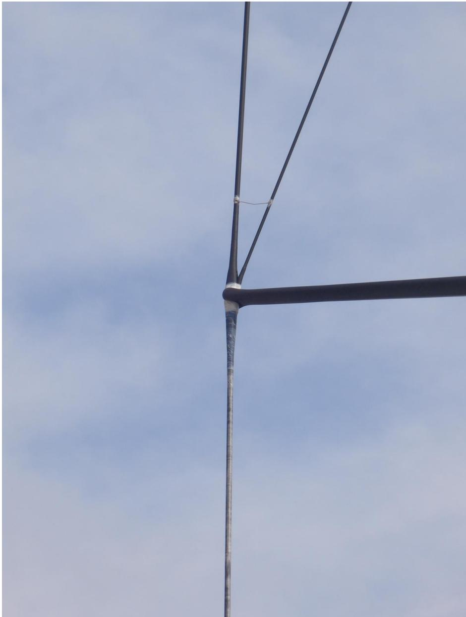
Fig 11: Spreader end detail with minimum bending moments in the cables and replaceable Diagonal.
